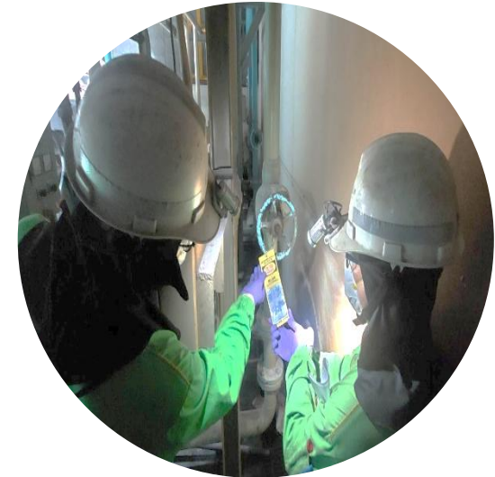
Pipeline equipment isolation & tagging for warning indication
