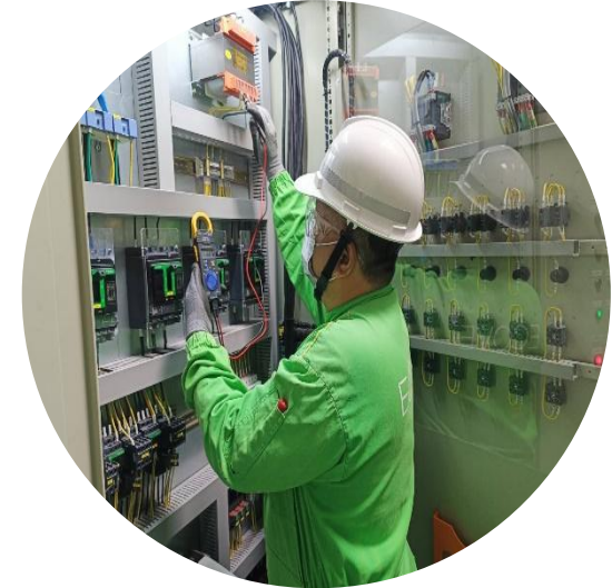
Power distribution panel inspection & maintenance
